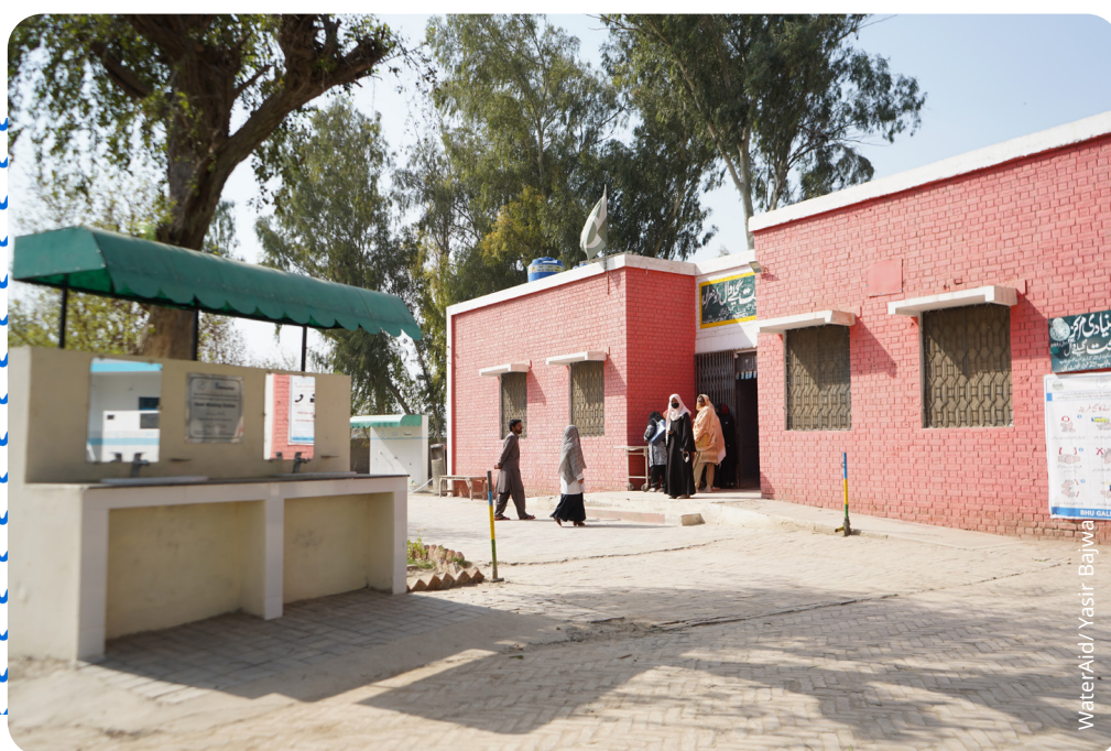
Handwashing station constructed by WaterAid in BHU Galleywal, District Lodhran, Punjab Province, Pakistan. March 2024
